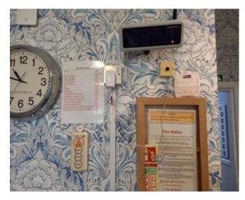
The home operates a call bell system, with display panels mounted on the walls at the reception area. The code for each room will show up on the small screen, so all staff can see it.
