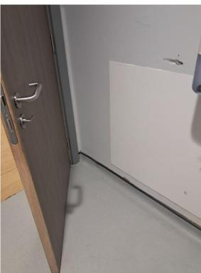
It was disappointing to note that even though the department had recently been refurbished there were already dents in the toilet walls, caused by the handles hitting the walls. Some form of stopper on the floor could prevent further cosmetic damage.
