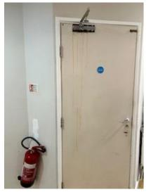
We noticed oil was running down from the hinge of one door in one of the corridors, and pointed this out to the activity coordinator.
