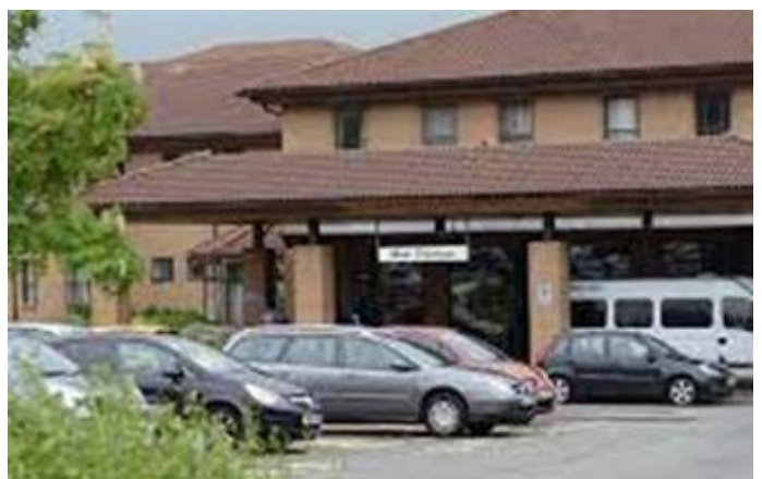
Princess Royal Hospital Telford
