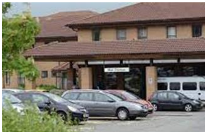
Princess Royal Hospital Telford
