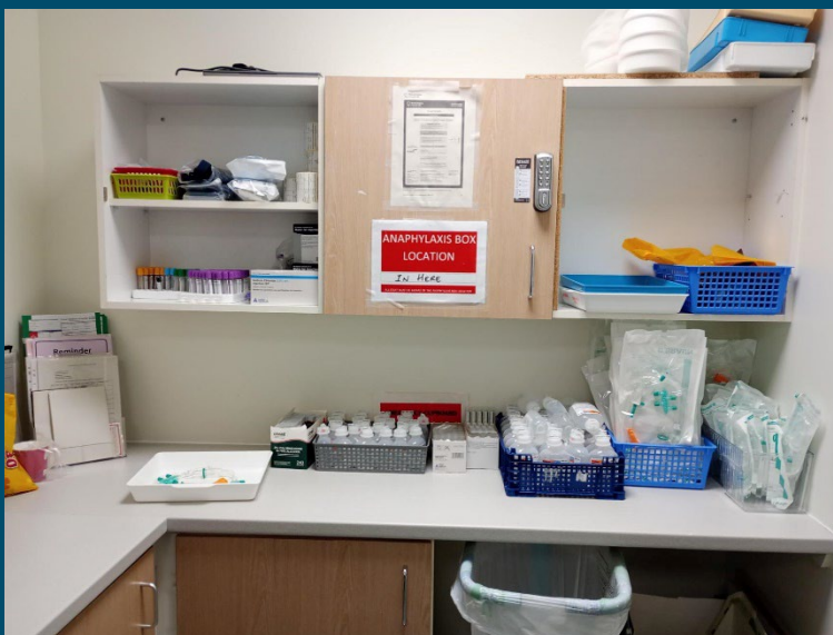
Broken cupboards in Coate ward.
