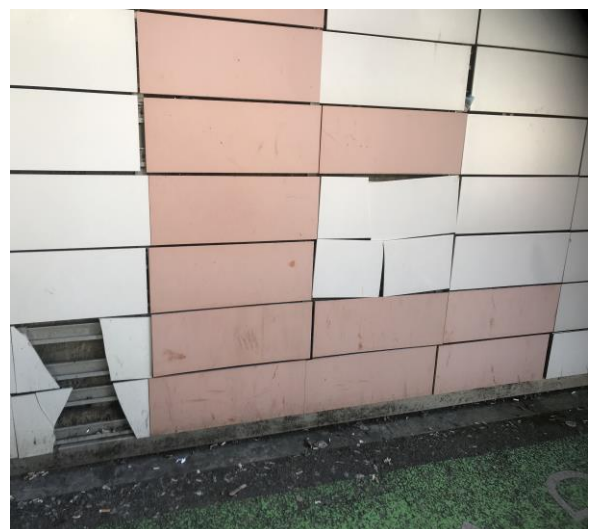
(Cracked cladding)
