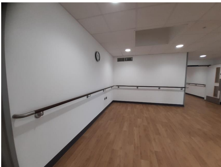
Grab rails line the centre corridors
