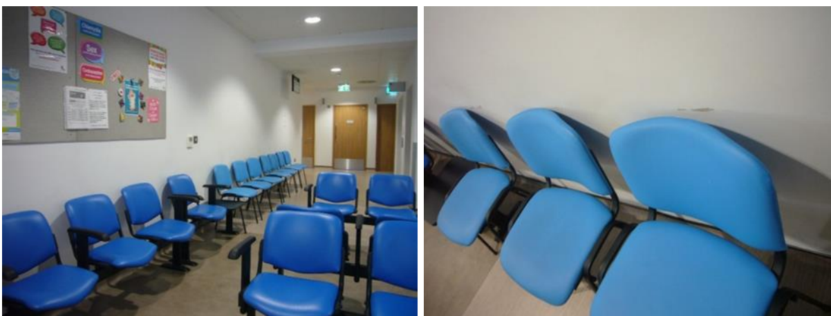
Fixed and not fixed (lighter blue) chairs - the latter damaging the wall.
