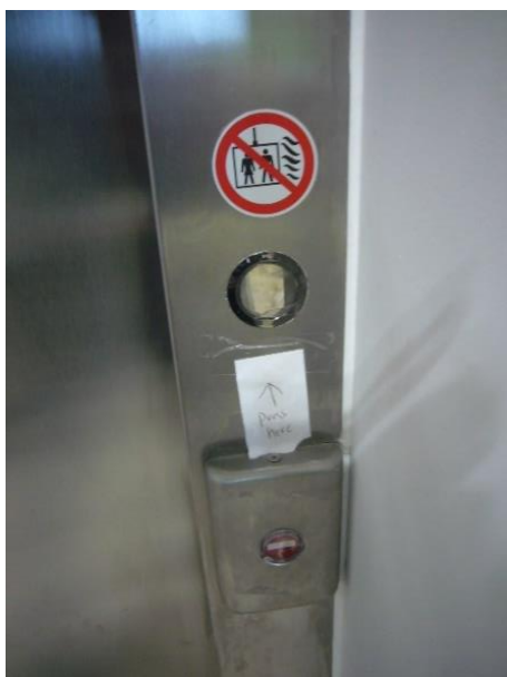
The signage on the lifts is confusing and has already resulted in a torn paper notice taped adjacent to the call button.
