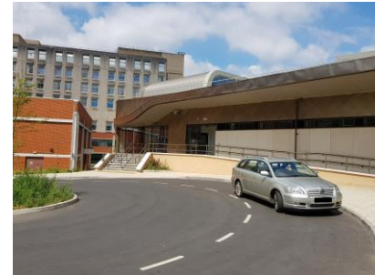
Figure 3 - Entrance to Emergency Department
