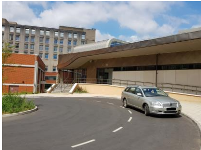
Figure 3 - Entrance to Emergency Department
